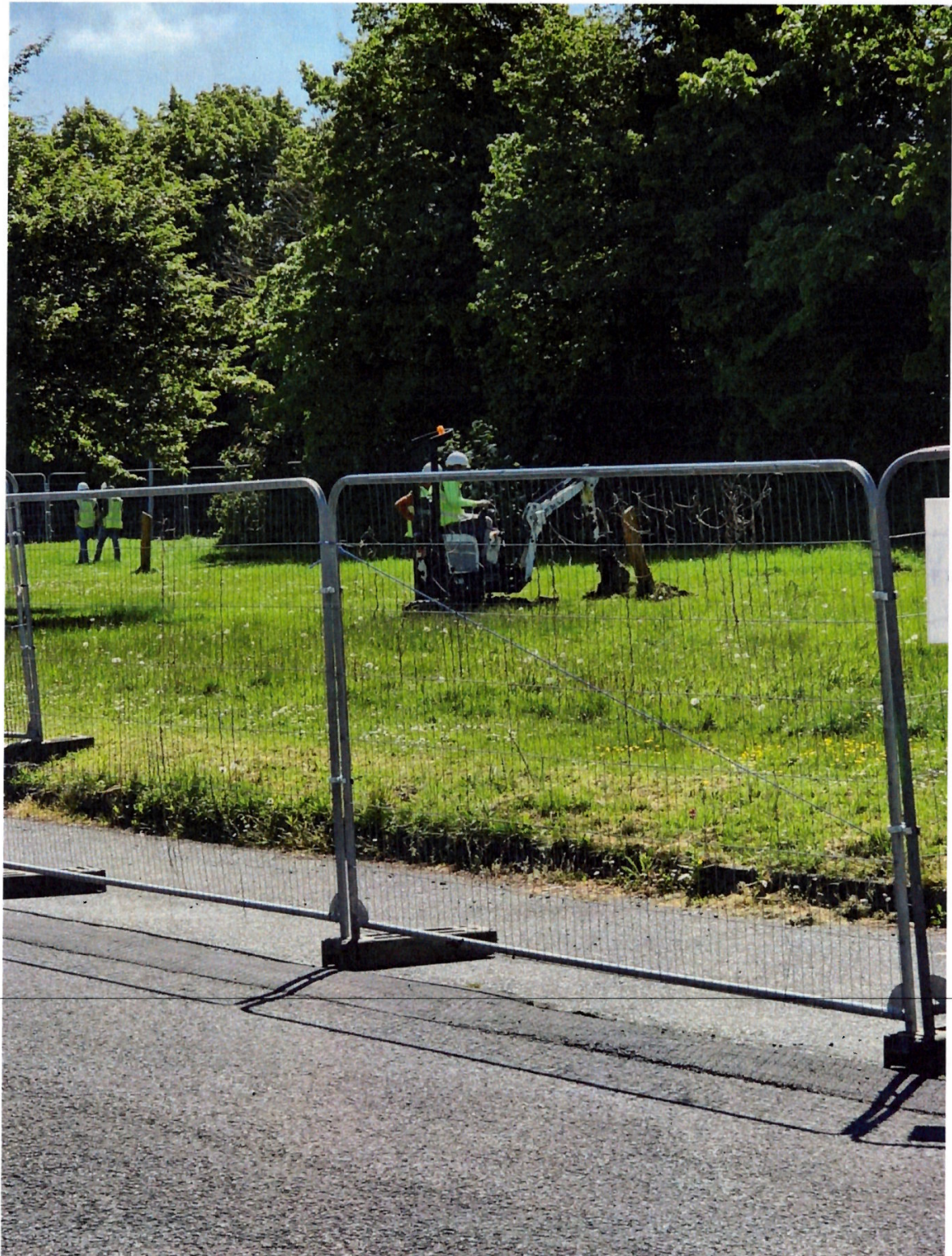
Kickabout posts being uprooted by mini-excavator
